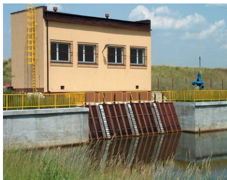
Fot. 7. Budynek pompowni nr 1 – widok po remoncie Phot. 7. Pumping station no. 1 – view after repair works
